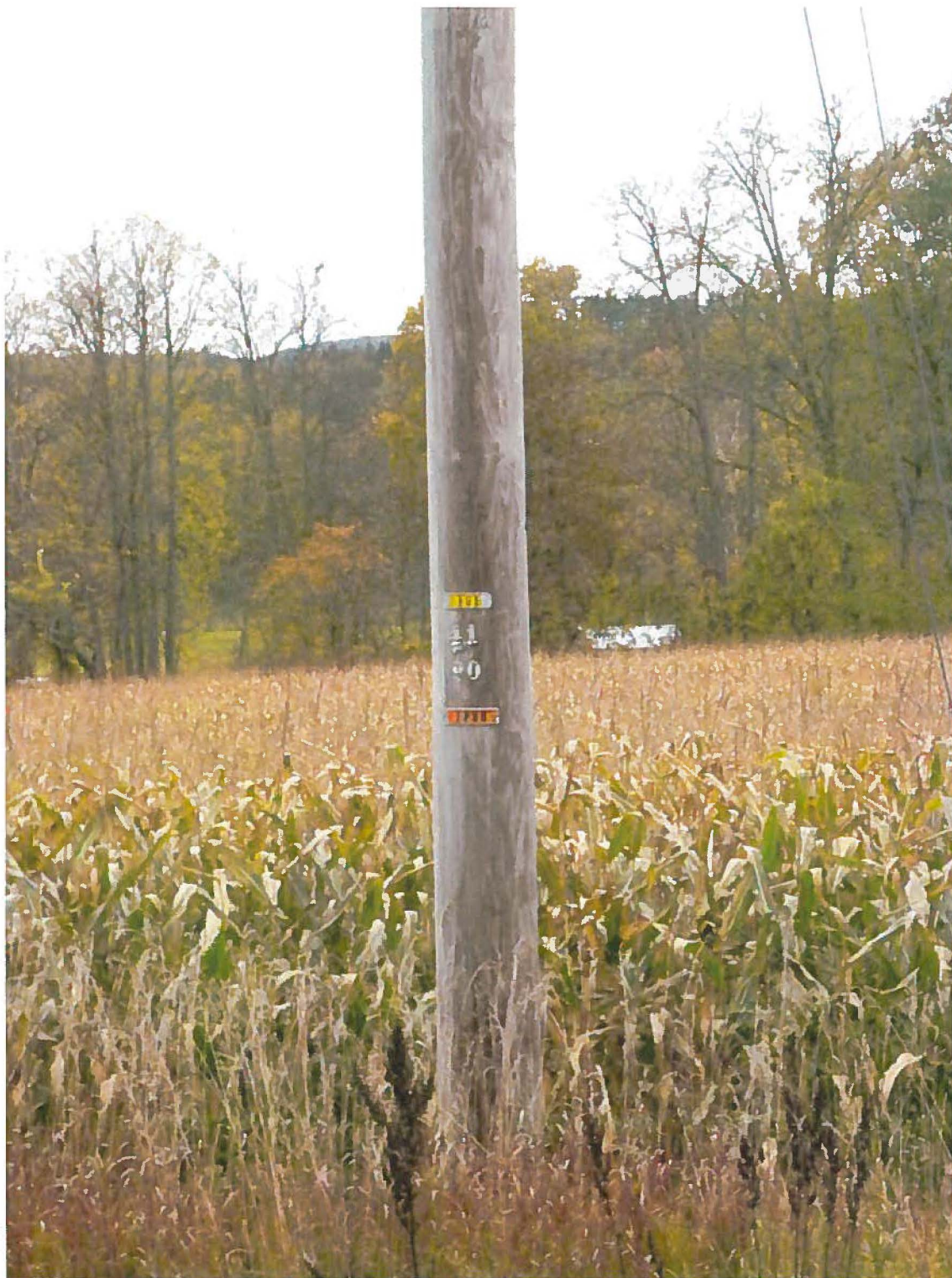
ORFORD NH Photo 2 of 4 Showing pole identification tags
